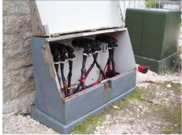
Figure 4.22 – Typical Junction Box
