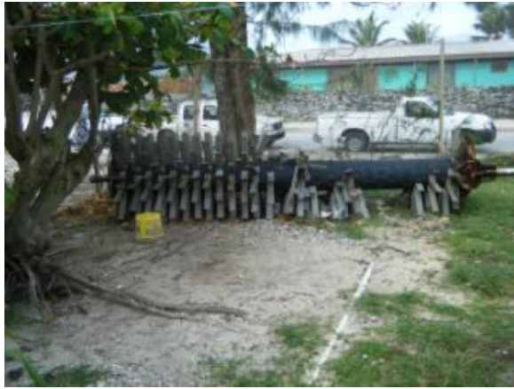
Figure 2.6 - Brush rotor removed and corroding
