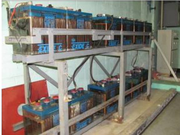
Figure 4.18 - Battery Cells
