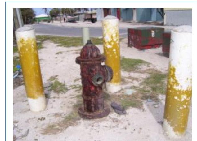
Figure 3.13 - Fire Hydrant Condition (typical)
