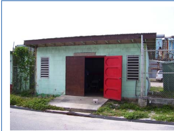
Figure 3.11 – SW Pump House 1 (typical)
