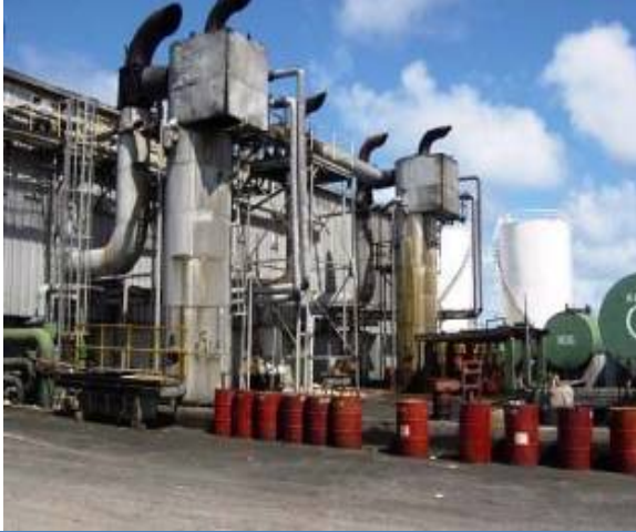
Figure 4.2A – West View of Power Plant
