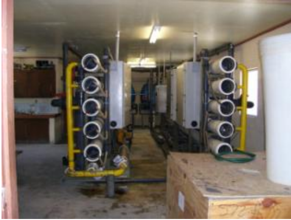
Figure 3.4 – RO1 and RO2 (100,000 gpd each)
