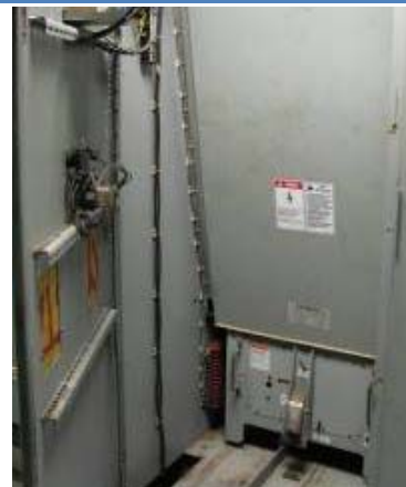
Figure 4.15 - Feeder Breaker
