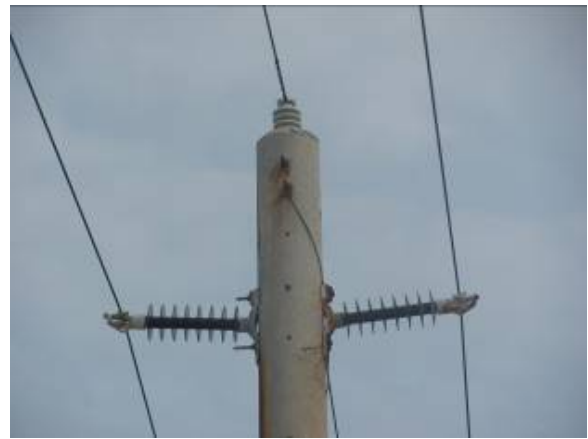
Figure 4.10 – Replace Pole Hardware Project
