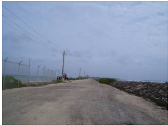
Figure 4.24 - Overhead Line Ebeye/Guegegue
