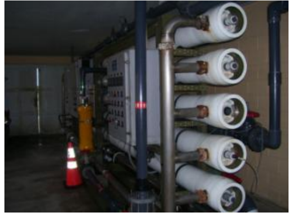
Figure 3.5 – RO1 and RO2 (100,000 gpd each)
