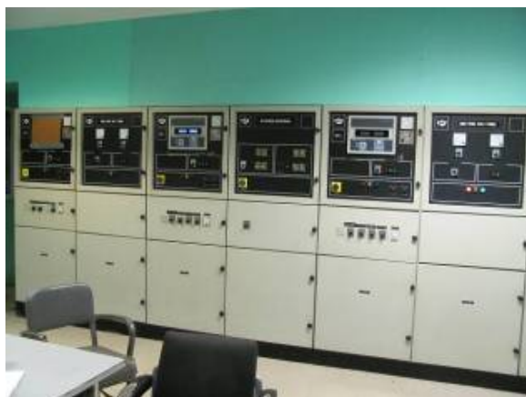
Figure 4.12 - Generator Switchgear
