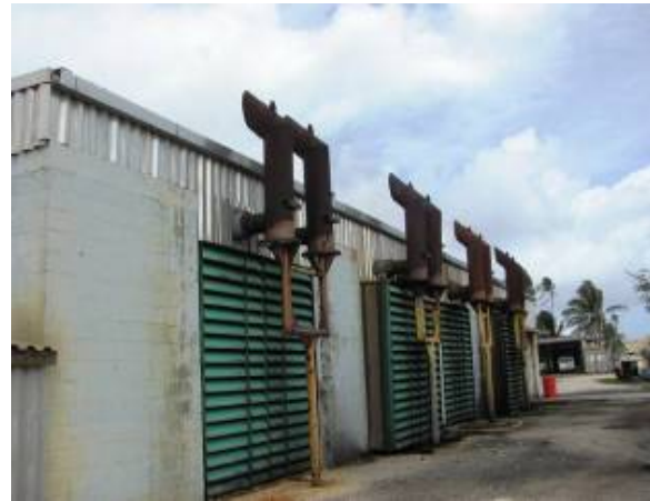
Figure 4.2B – East View – Smokestack System
