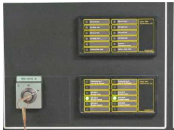
Figure 4.13 - Typical Generator Control Panel
