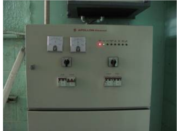
Figure 4.19 - Charger/Rectifier
