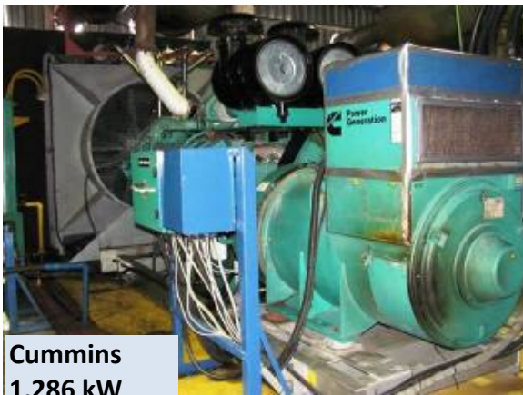
Figure 4.5 - Diesel Generator #2
